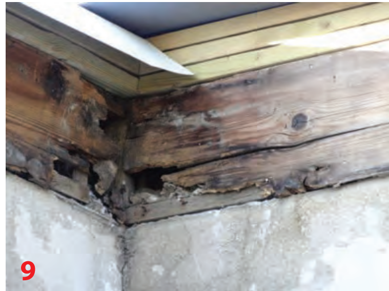
FLAGLER COUNTY PROVIDED PHOTOS OF ROTTEN WOOD AREAS
