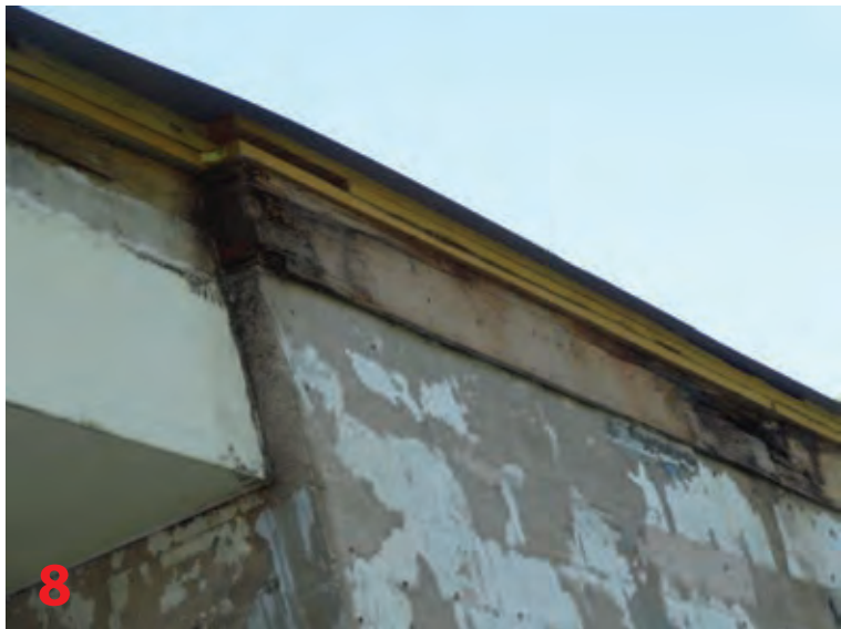
FLAGLER COUNTY PROVIDED PHOTOS OF ROTTEN WOOD AREAS
